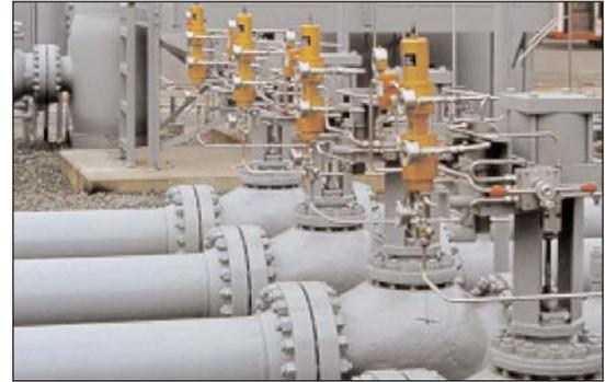
**Figure 8.0** - Becker Model VRP-Pilots on Globe Valve Regs
