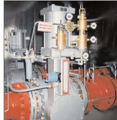
**Figure 9.0** - Becker Model VRP-Pilots on Ball Valve Regs
