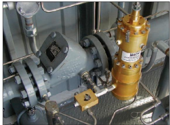
**Figure 10.0 - Becker Model FEP-1300-CH Flexflo® Pilot**
