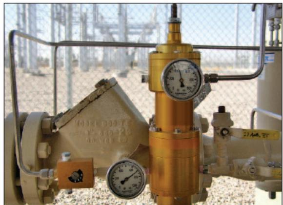
**Figure 11.0 - Becker Model FEP-600-CH Flexflo® Pilot For Power Plant Fuel Gas Regulation**
