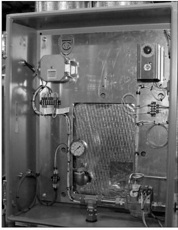
(Figure 4.1.4.d) Control box for a CWT385 Vacuum Boiler.
