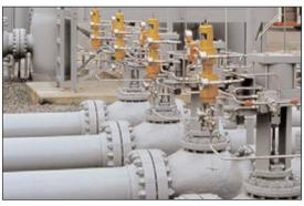
Figure 8.0 - Becker Model VRP-Pilots on Globe Valve Regs Becker VRP-Pilots combined with Becker LPDA Series Actuators used on globe pattern valves are ideal for regulation in LDC systems. Incorporation of the BPS $^{\text{TM}}$  feature eliminates all atmospheric emissions.
