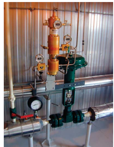
Figure 8 - VRP-SB-CH Retrofit Virtually Eliminates Atmospheric Bleed Gas
