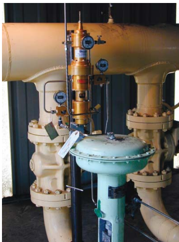
Figure 7 - VRP-SB-CH Retrofit Simplifies Control Instrumentation
