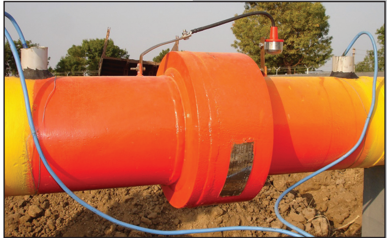
Installed Pipe Pup in the field.
