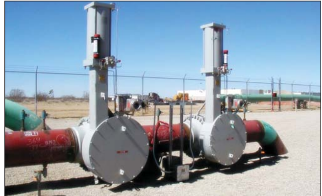
Figure 9.0 - Becker Model DNGP Electro-Pneumatic Positioner on Large Bore Ball Type Control Valves
