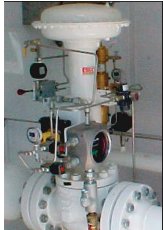
Figure 11.0 - Becker Model DNGP Positioner Retrofit to Other Manufacturer's "Vee" Type Control Valve
