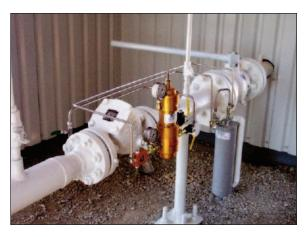
Figure 11.0 - Becker Model FEP-600-CH Flexflo® Pilot For Power Plant Fuel Gas Regulation
