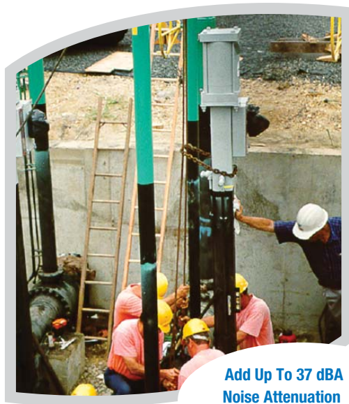
Figure 6.0 - Installation of Becker Below Ground Ball Valve Regulator.
