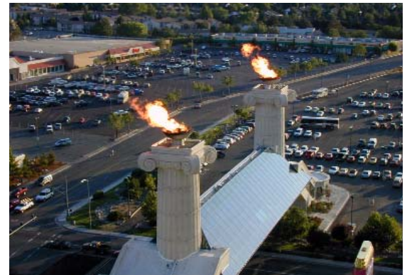
Figure 14.0 - Flame On! Becker Globe Type Control Valves provide pressure regulation for control of natural gas "torches" constructed at a popular Reno, Nevada casino. See Figure 15.0 for additional information.
