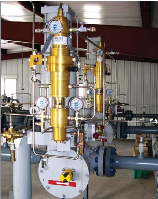
Figure 8.0 - Becker VRP-SB-PID Installed On A Becker Ball Valve Power Plant Monitor
