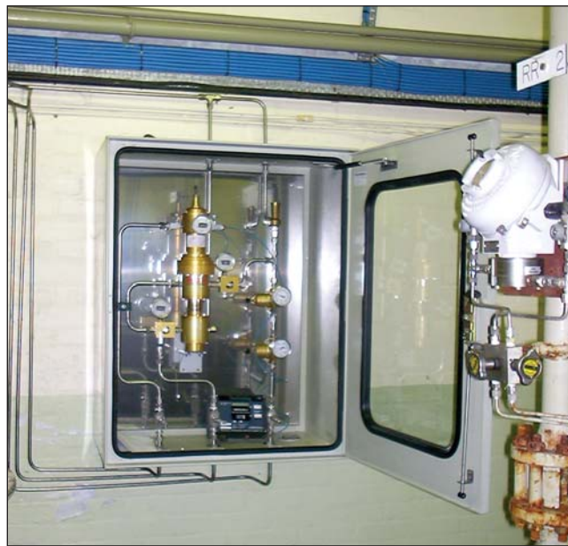
Figure 7.0 - VRP-SB-PID Retrofit to "Jetstream" Regulator
