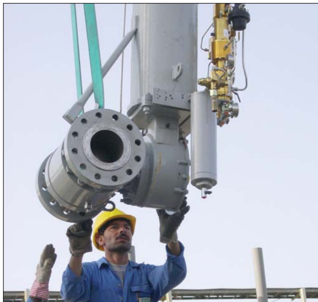
Figure 6.0 - VRP-SB-PID For Underpressure Protection
