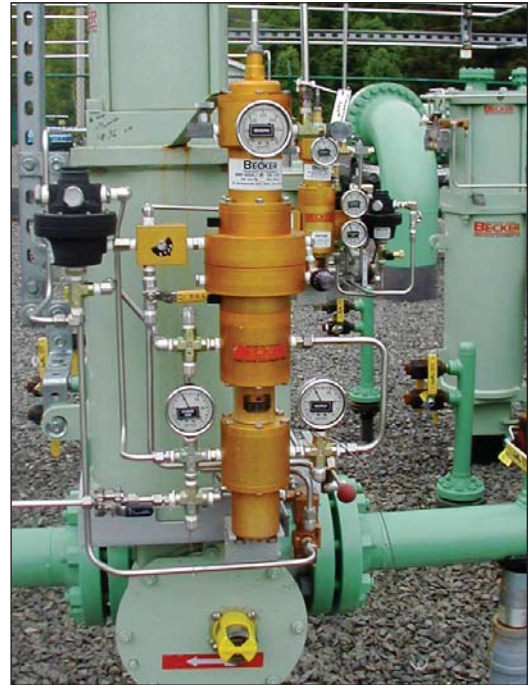
Figure 17.0 - Becker Ball Valve Power Plant Regulator Utilizing The Becker VRP-SB-PID
